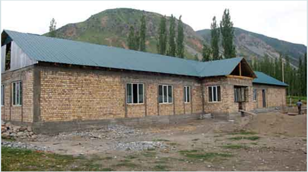
A school under construction with SDC support
